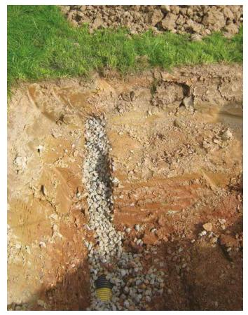
Figure 34. Permeable backfill in trench over drain
