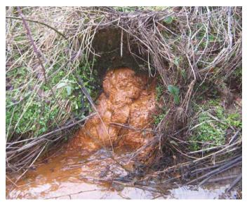
Figure 24. Drainage outfall blocked by ochre
