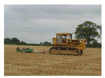
Figure 30. Installing mole drains
