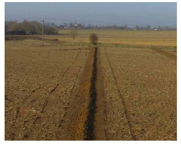
Figure 29. Recently installed drains
