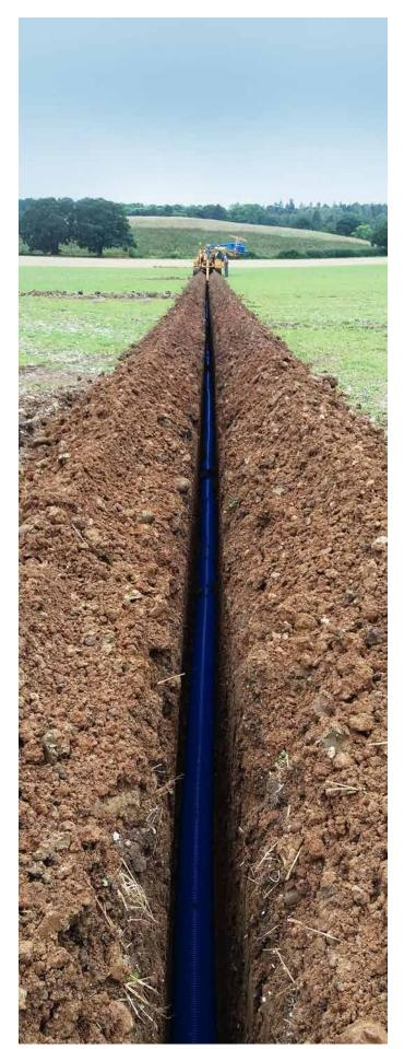
Figure 32. Install drains at an appropriate depth and constant gradient (fall)
