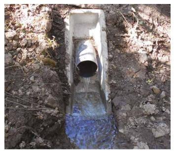
Figure 38. Precast concrete headwall (type K)
